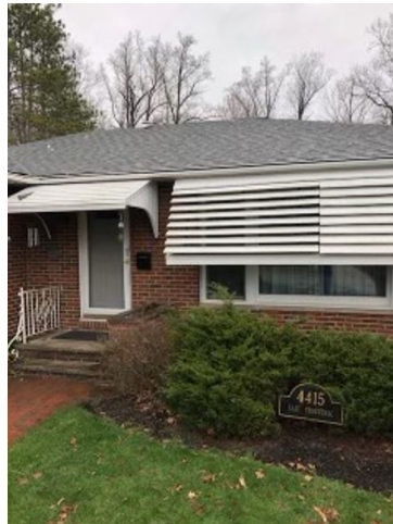
4415 East Frontenac, front view.
